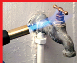
Thawing frozen pipes
